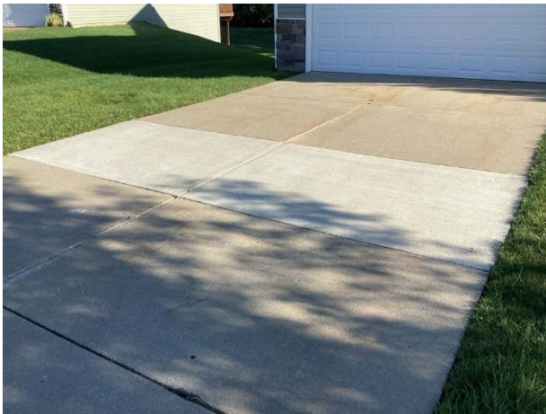
Replaced section of driveway
