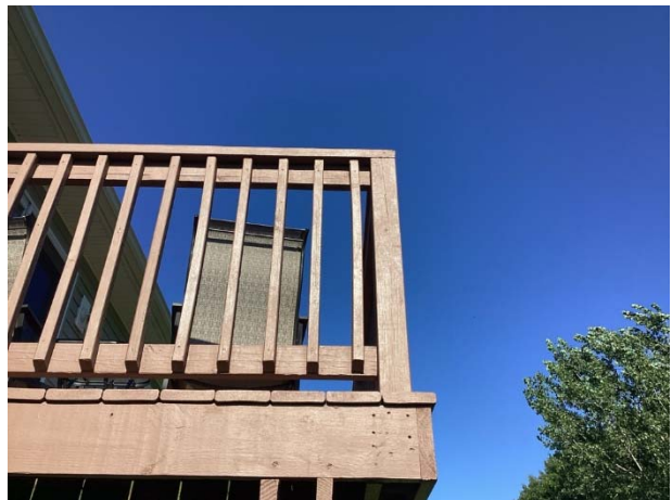
Warped baluster
