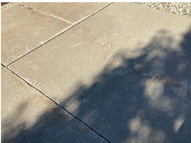
Driveway cracks
