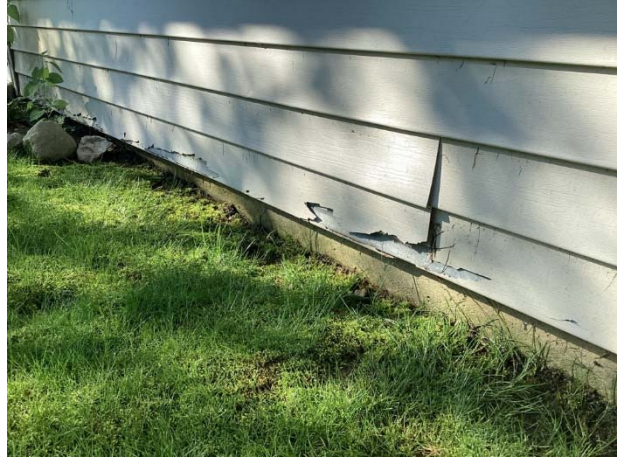
Siding damage
