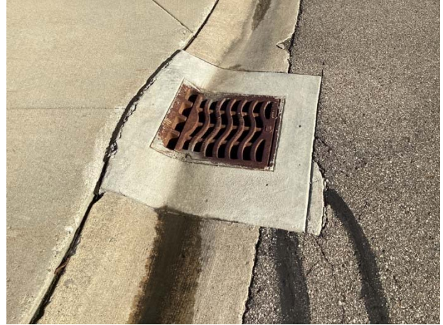
Catch basin repair
