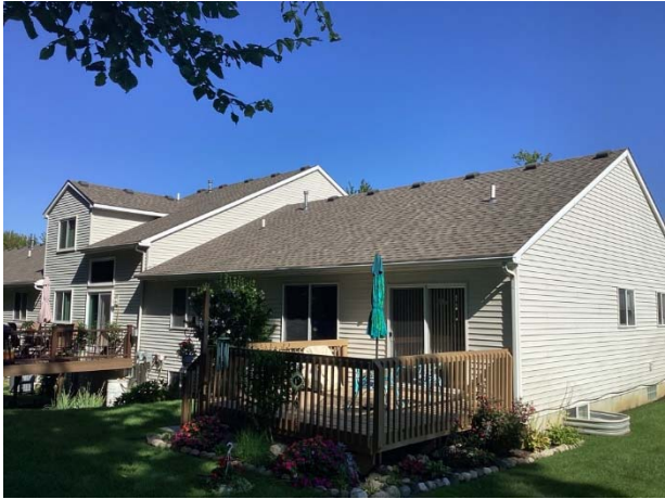
Roof overview (previously replaced)
