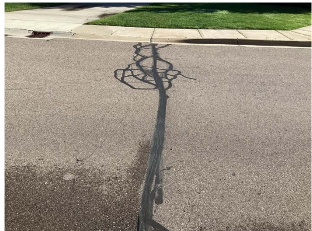
Pavement cracks
