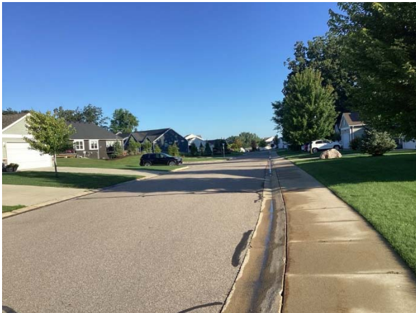
Pavement overview (Yarrow shown)
