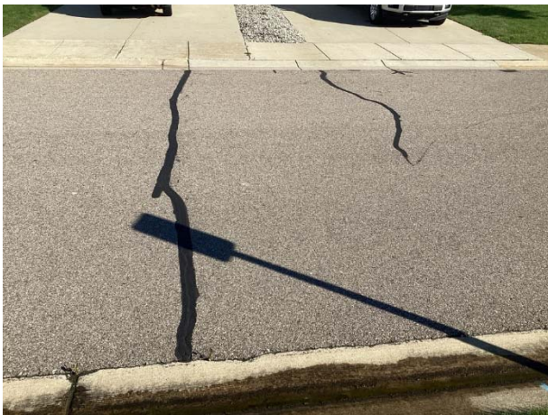
Crack repairs
