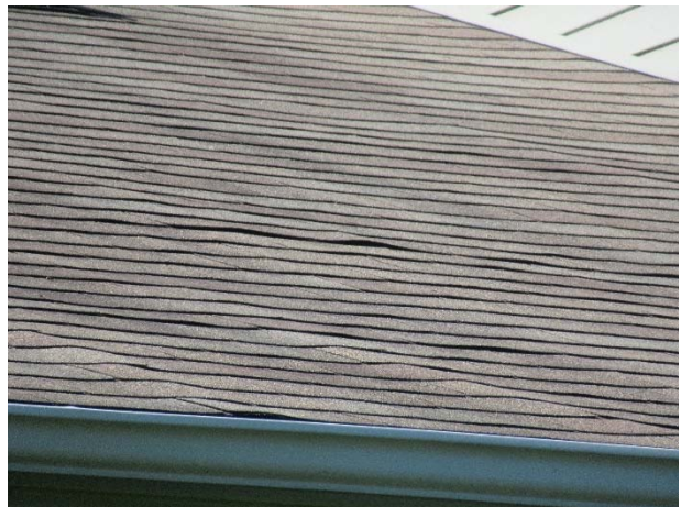
Shingle lift (112 Sedum Road shown)
