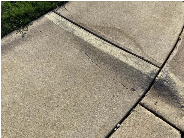
Sidewalk cracks
