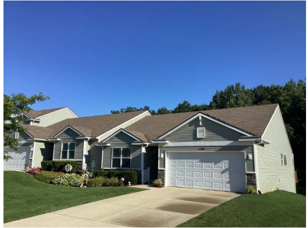
Roof overview (original)
