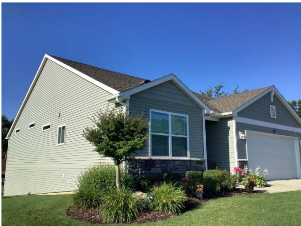
Vinyl siding overview
