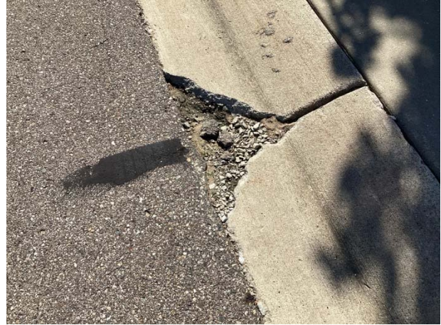
Concrete spalls
