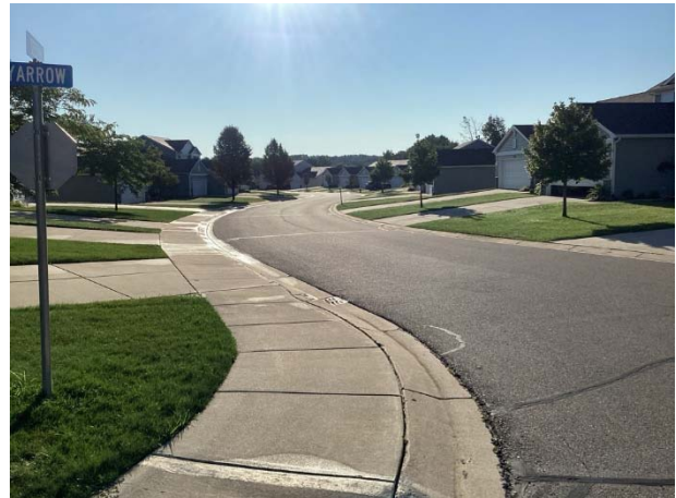
Pavement overview (Sedum Road shown)
