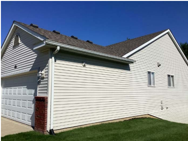
Aluminum gutters and downspouts
