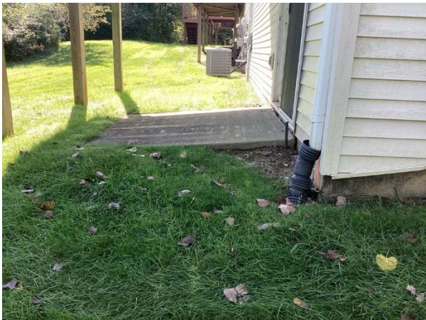
Patio settlement (1012 Spirea shown)
